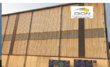
↑ After 10 Year, 2021 No Corrosion & No Other damages
