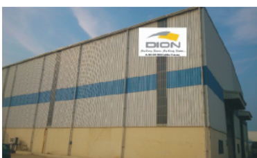
↑ 125000 sq.ft. (approx) project done in the year 2011 Galvanizing Plant 3.0mm Thickness for Roof 2.00mm Thickness for Wall
